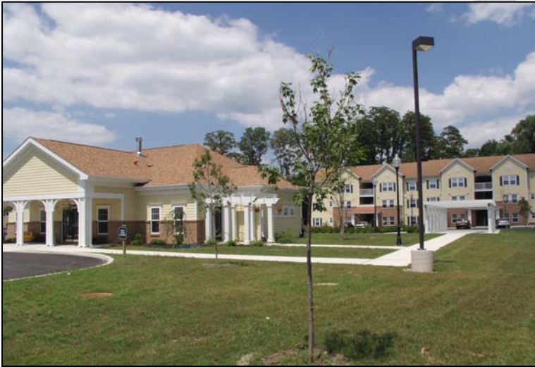
A new senior housing complex in the Town
